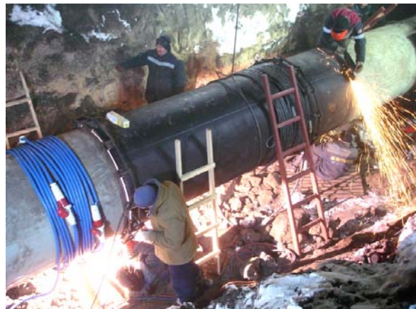
Fig. 9. Repair works on the main gas pipeline DU 1200×12 mm «Urengoy-Pomari-Uzhgorod» using the technology of demagnetization of welding joints developed at the ITPM of the National Academy of Sciences of Ukraine (Ternopil, 2017)
